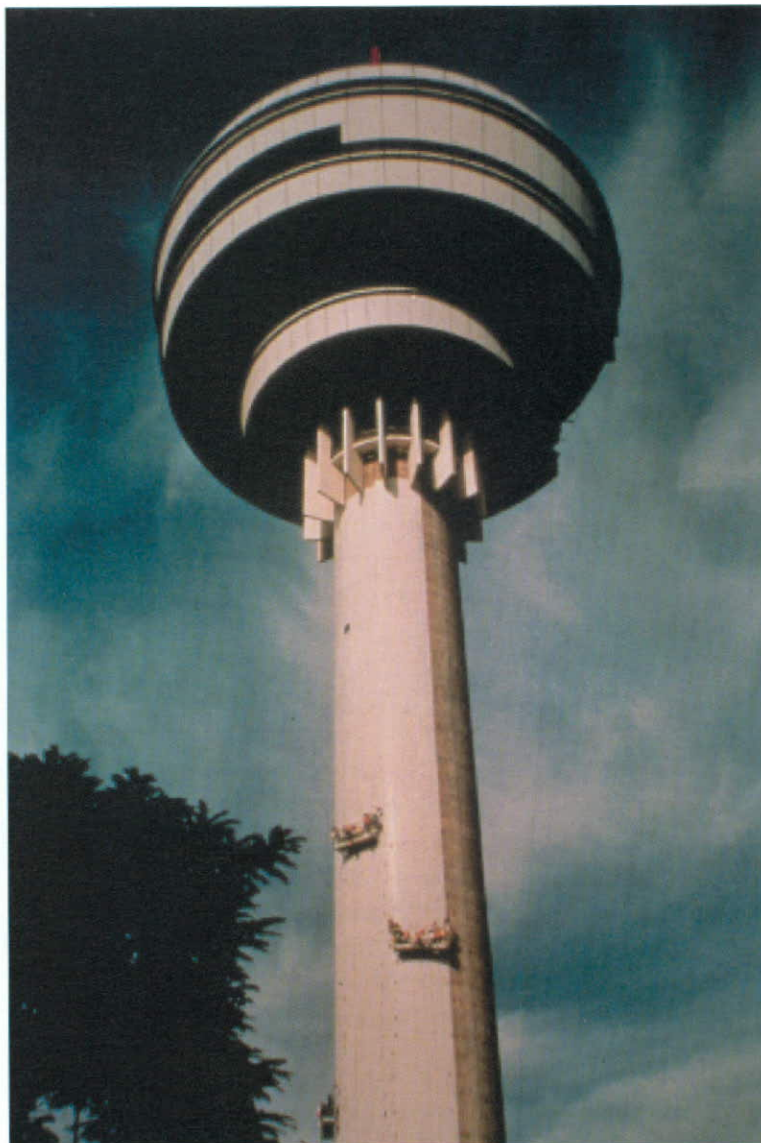
The Tele Diffusion Tower in Paris, France, is 160 meters high, the tallest, occupied, slip-formed concrete structure in Europe. Each story of the tower consists of approximately 1,200 tons of precast concrete faced with ceramic tile.
