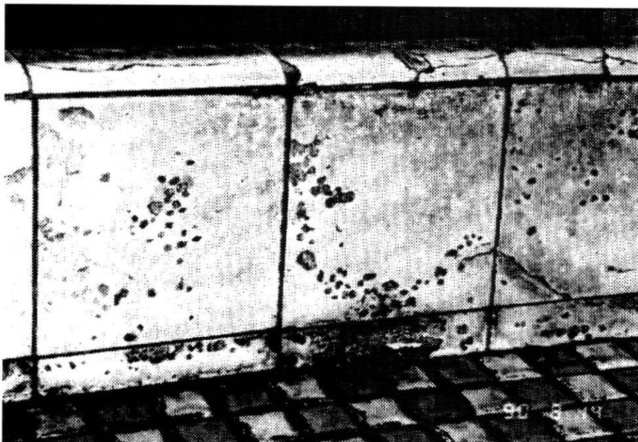
Fig.1 Frost damage in the case of interior tiles of a bathroom
