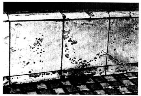
Fig.1 Frost damage in the case of interior tiles of a bathroom
