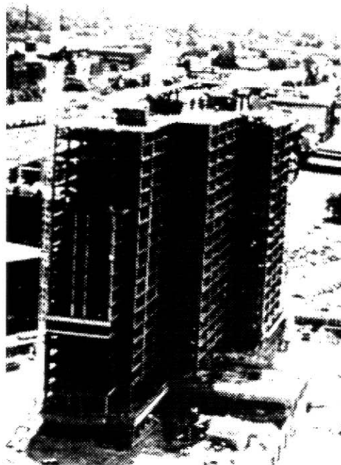
FIGURE 2 SKELETAL STRUCTURAL FRAMING SYSTEM
