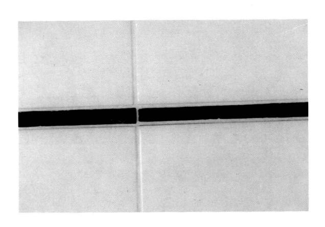
Photo 7.-If the tiles are set according to the projections of the relief, the piece will be set more deeply than required.
