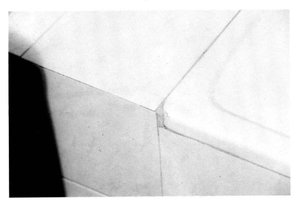
Photo 10.-The point where the bathtub meets the dihedral angle produces the inevitable triangle with one curved edge
