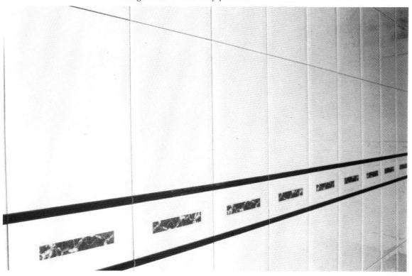
Photo 12.-Designs like this one make it possible for the listel and the most projecting parts of the tile work to be on the same plane.
