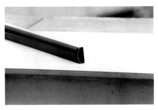
Photo 13.- Listels which project from the flat plane of the tile work make corner joints difficult.
