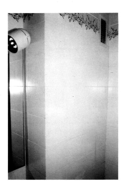
Photo 3 bis.-The heterogeneity of the base is one of the causes of tiles comi
