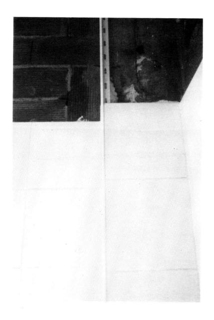
Photo 17.-The adhesive material permits the raising of ceramic tiles to the same level as the edge of the corner bracket. If this is not the case, surface continuity will not be true.
