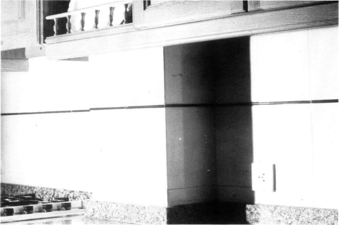
Photo 3.-The existence of buttresses in a wall makes tiling difficult.
