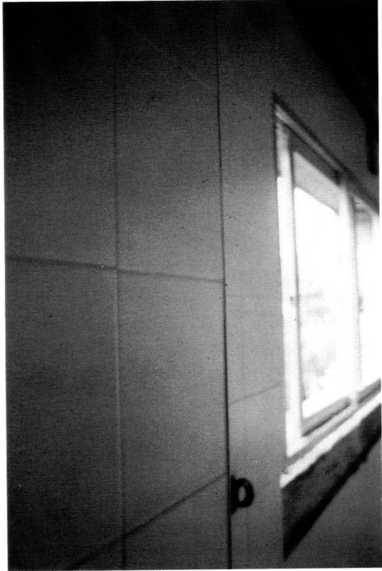
Photo 16.-Finishing touches such as this corner bracket must be correctly lined up in order to achieve continuity and tangence between the sides of the angle.
