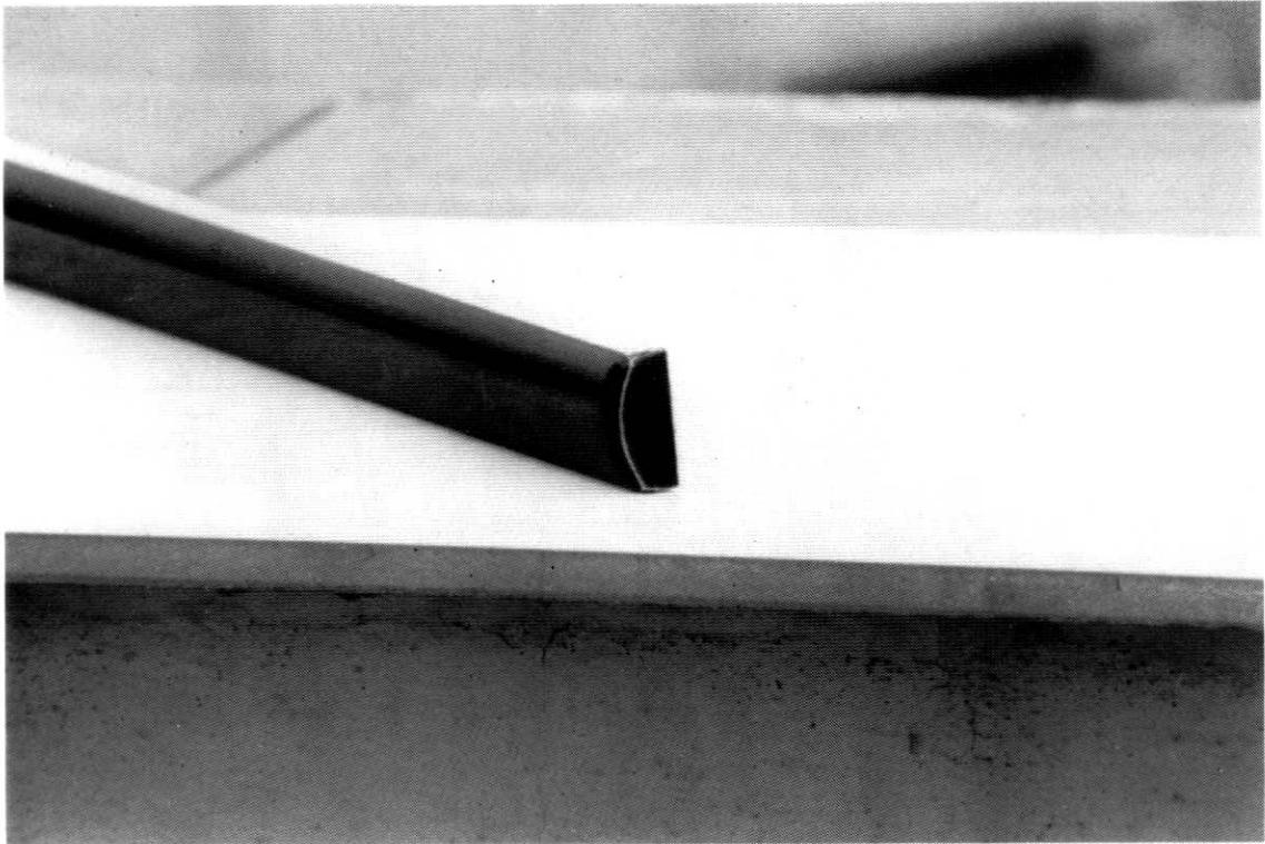
Photo 13.- Listels which project from the flat plane of the tile work make corner joints difficult.
