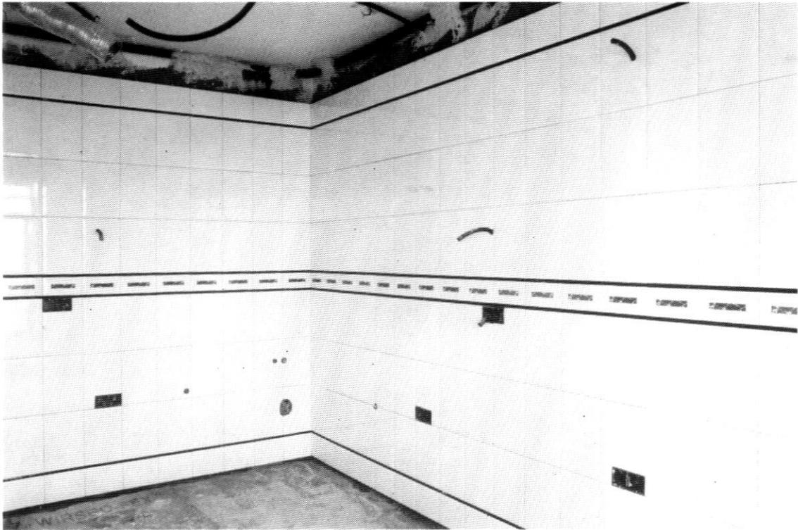
Photo 11.-The joins between the tiled area and the fixtures and fittings must be carefully planned in advance.
