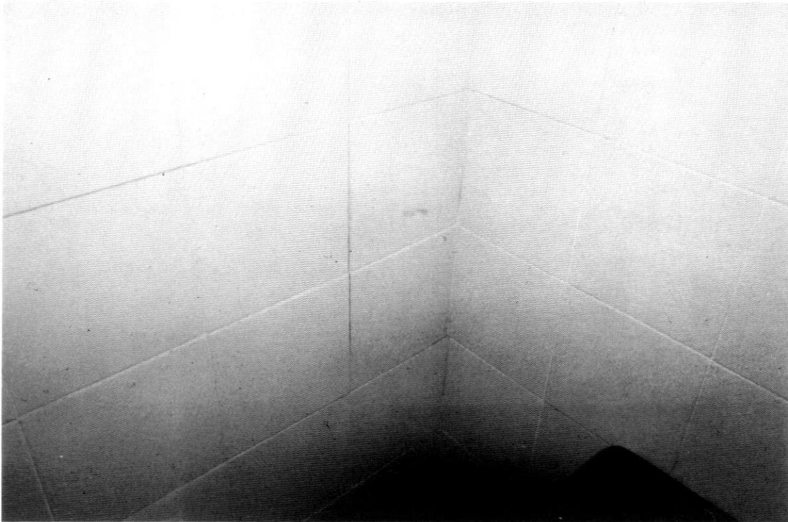
Photo 4 bis.-Tiling over a base lacking in due stability can in the future cause tiles to be displaced, as is the case with this tiling job, done a ventilation duct
