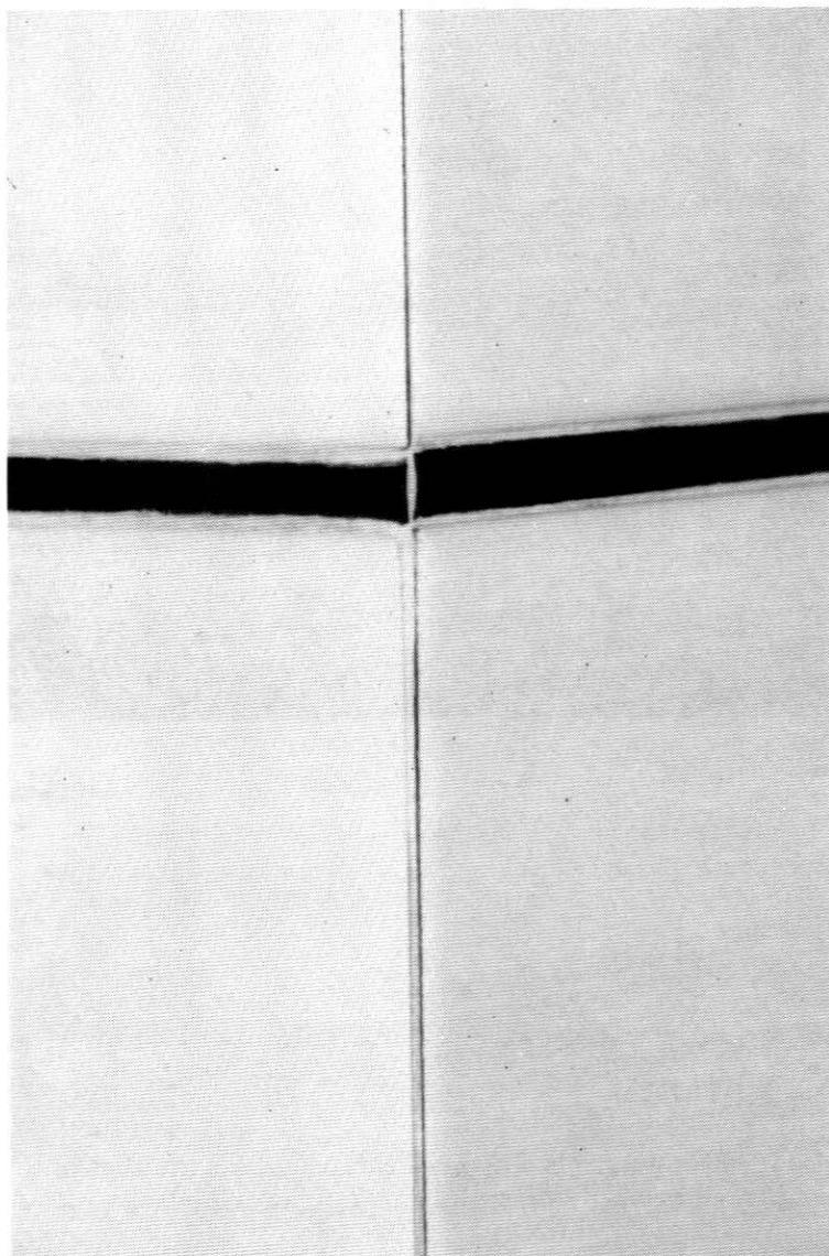
Photo 5.-Defects in corner joints affect the overall quality.
