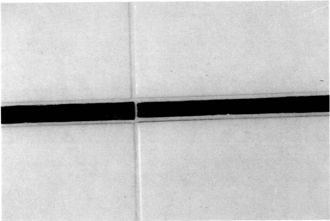
Photo 7.-If the tiles are set according to the projections of the relief, the piece will be set more deeply than required.
