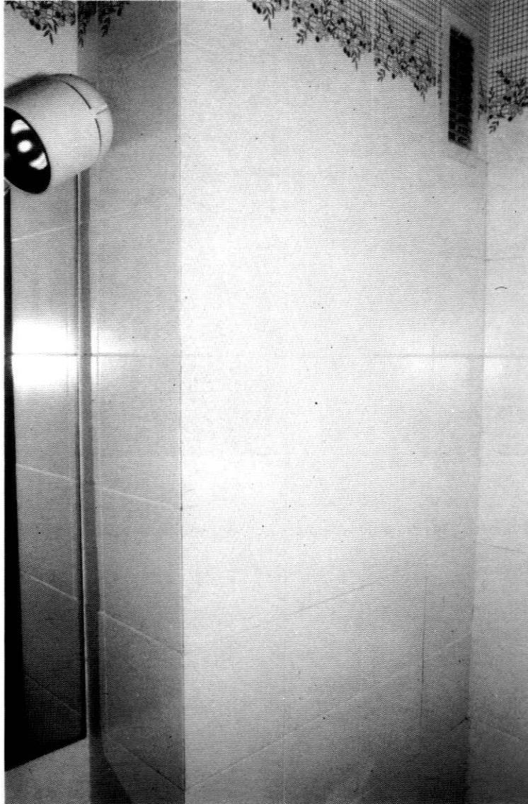
Photo 3 bis.-The heterogeneity of the base is one of the causes of tiles coming
