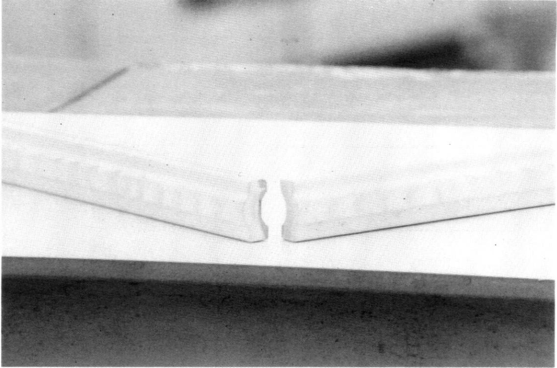
Photo 6.-The relief in the listels makes it more difficult to achieve a flat surface and neat joints.
