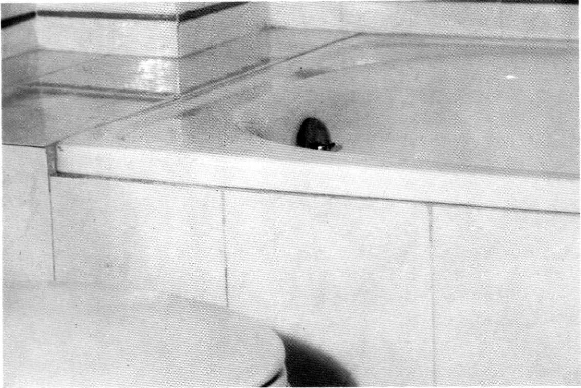
Photo 9.-The join between the lap and the bathtub is often difficult.
