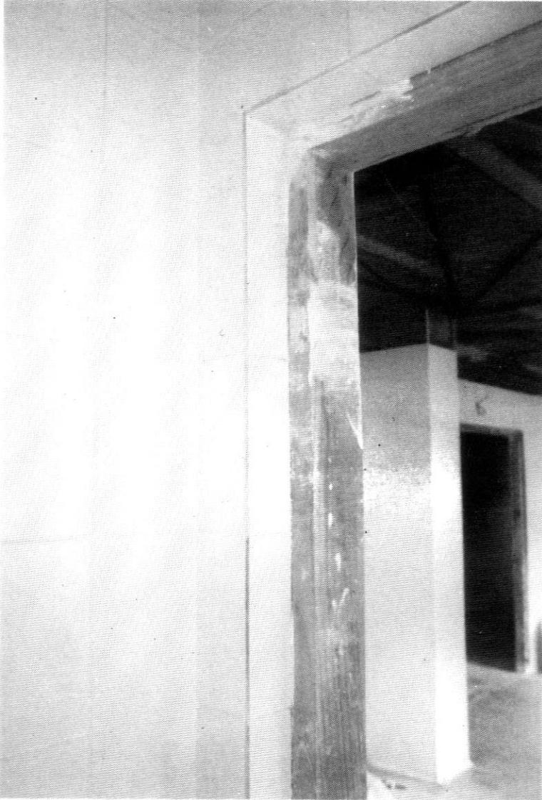
Photo 15.-Tiling which leaves the biscuit base of the tile visible, as in the case of this corner, does not offer even the most elemental level of quality.
