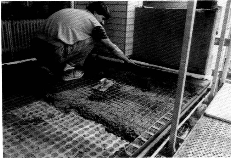
Fig. 9: Working with a surface drainage system
