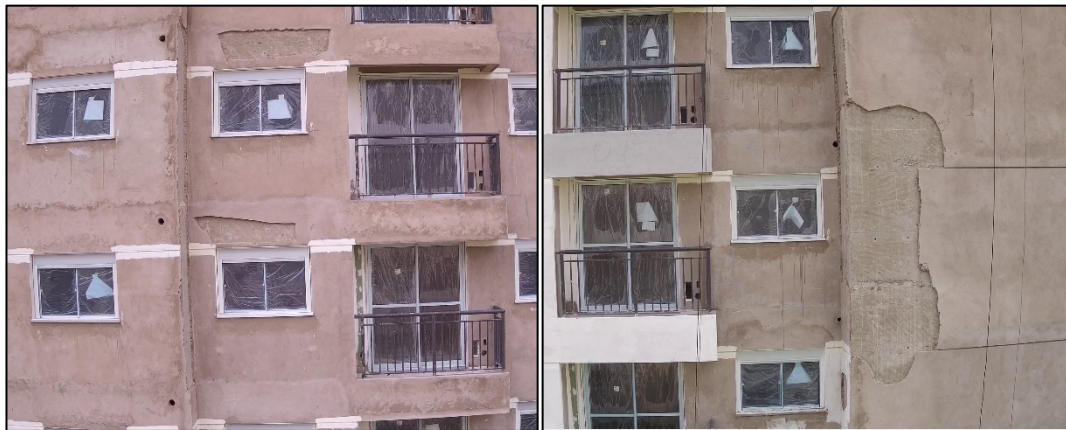
Figure 3 – Pathological manifestation of detachment at the covering interfaces with the concrete surface, even during the execution phase of the adhered covering system.
