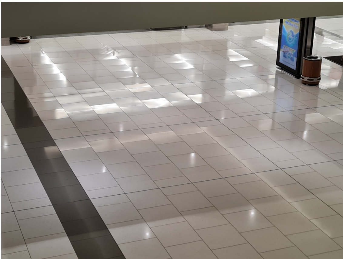
Photograph 3 -Stone tile flooring which has cupped and curled in a commercial shopping centre.
