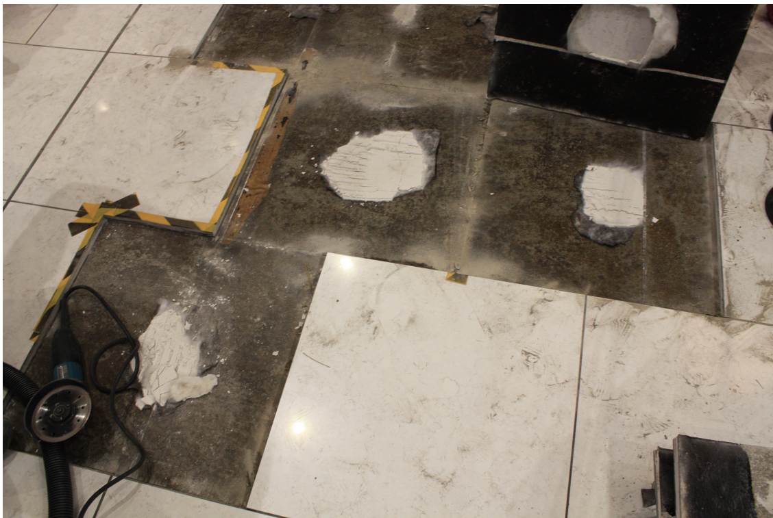
Photograph 4 -Engineered stone tile installed on a crack suppression mat and subsequently curled and partially delaminated.
