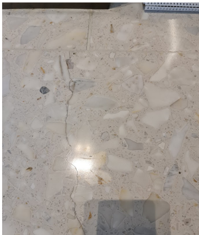
Photograph 1 -Commercial shopping centre cracking in quartz tile at a cold joint location.
