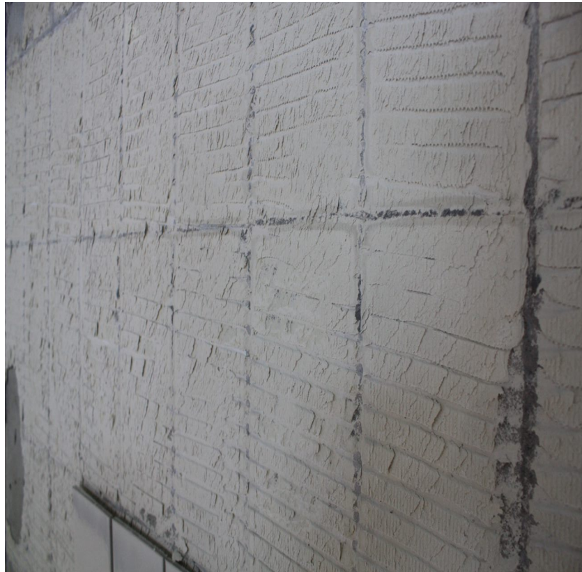
Photograph 5 – shows evidence shear forces on the tile adhesive inside a pool where failure has occurred.
