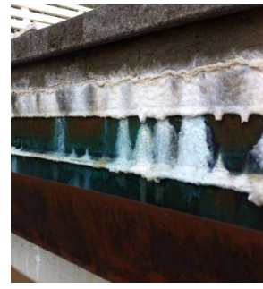
Screed weakening as a result of water percolation.
