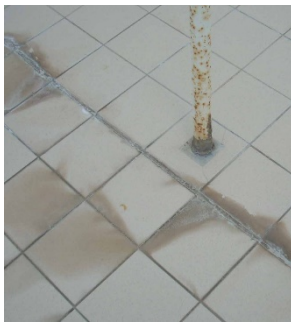
Formation of salt efflorescence and mould in joints.
