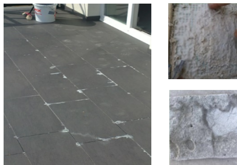
Figure 5. Effects of alkaline hydrolysis on ceramic flooring
