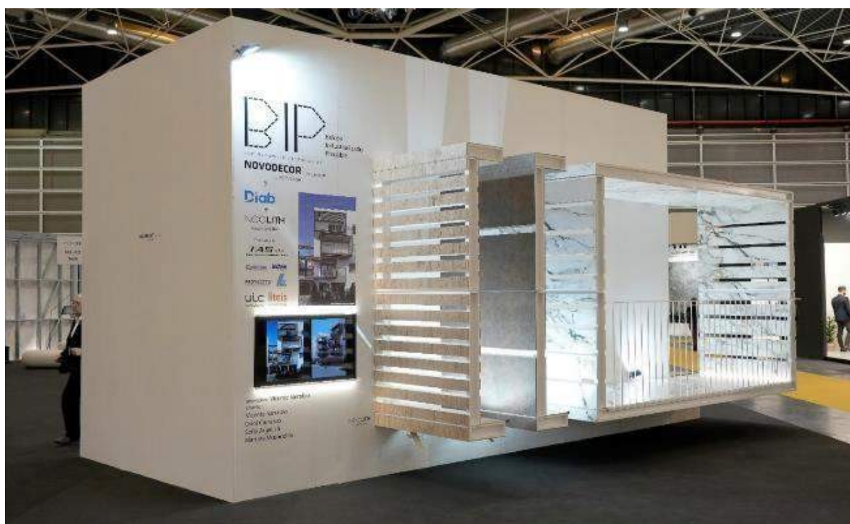
Figure 23. Photo of the folding industrialised balcony (FIB) prototype, Cevisama 2023, clad with porcelain tile, thanks to the structural ceramic sandwich.
