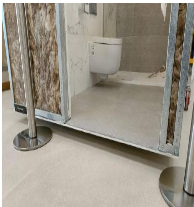
Figure 16. Photo of a ceramic sandwich on an industrialised bathroom floor (1.2 cm).
