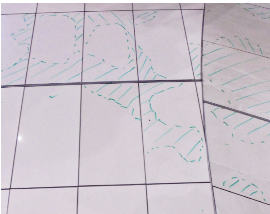
Figure 3. The repeat mark-up by a different operative about a year later, taken without reference to the first photo found a slightly greater area of hollow tiles. This could indicate that the hollowness is expanding, or it could just be operator variation in perception or equipment used. Either way the assessment of the hollow sounding areas has been made more valid and reliable because it can be repeated. This is good but not perfect.
