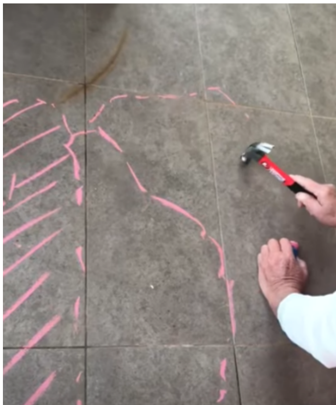
Figure 1. Here a small hammer and chalk are used to mark out the drummy area.
